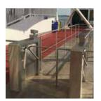
A full height Boon Edam Turnlock 100 turnstile allows for **easy departure** while presenting a **visual deterrent** and **preventing unauthorized access** back to the Ferris wheel.
